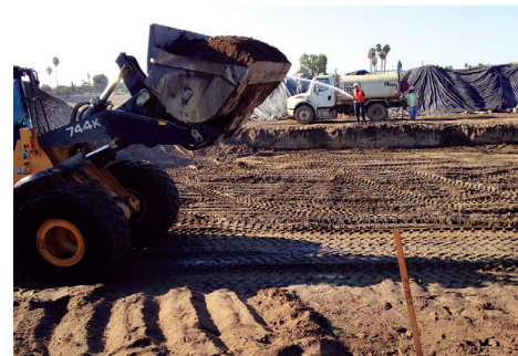
Backfilling of Excavated Area
